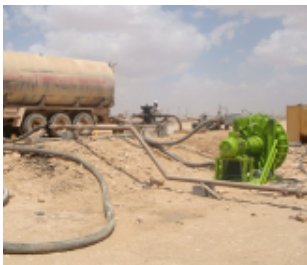
ALH125 crude oil pumping
